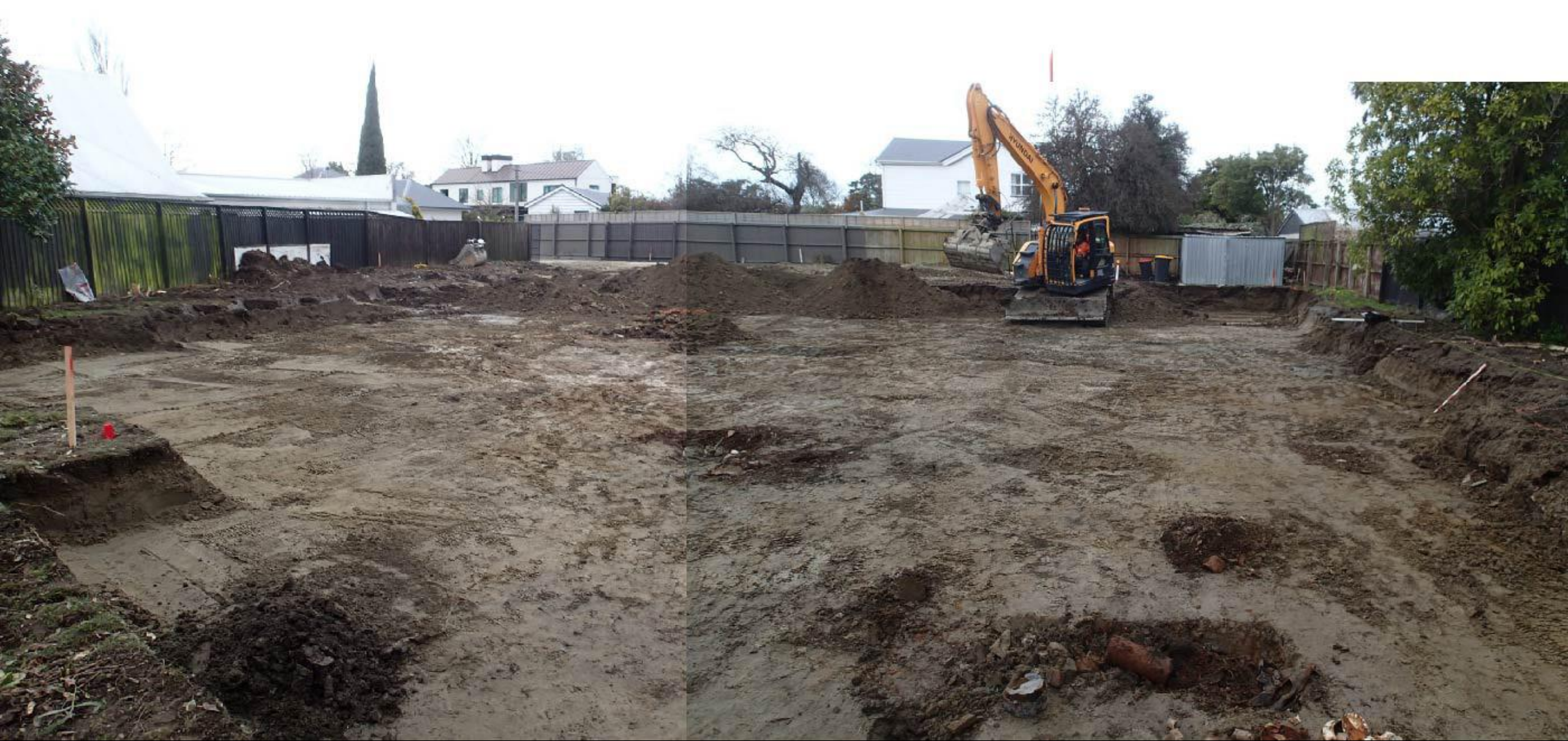
Earthworks monitoring complete.
